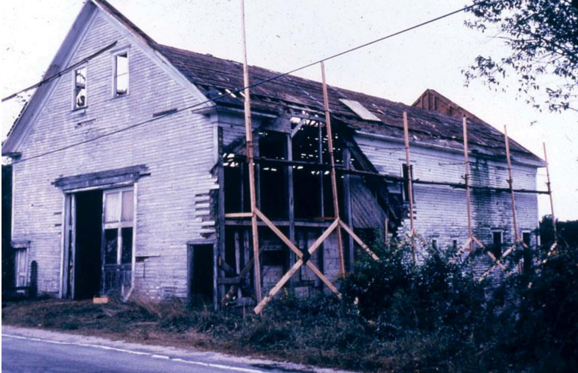
The Performing Arts Center is actually composed of two barns. The smaller barn, now on left facing side of the PAC, originally was attached to the right facing side of the larger barn, pictured here.
