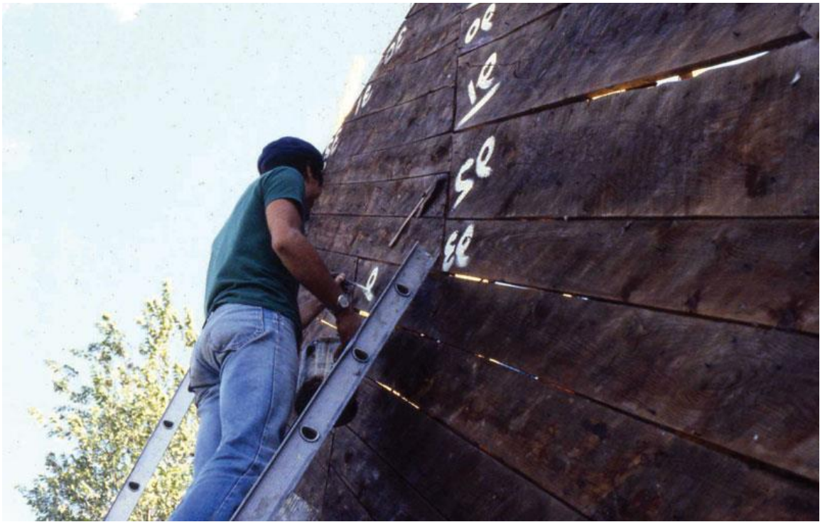
Students meticulously numbered every architectural element (including clapboard, beams, posts, and, here, sheathing) to ensure proper reassembly.
