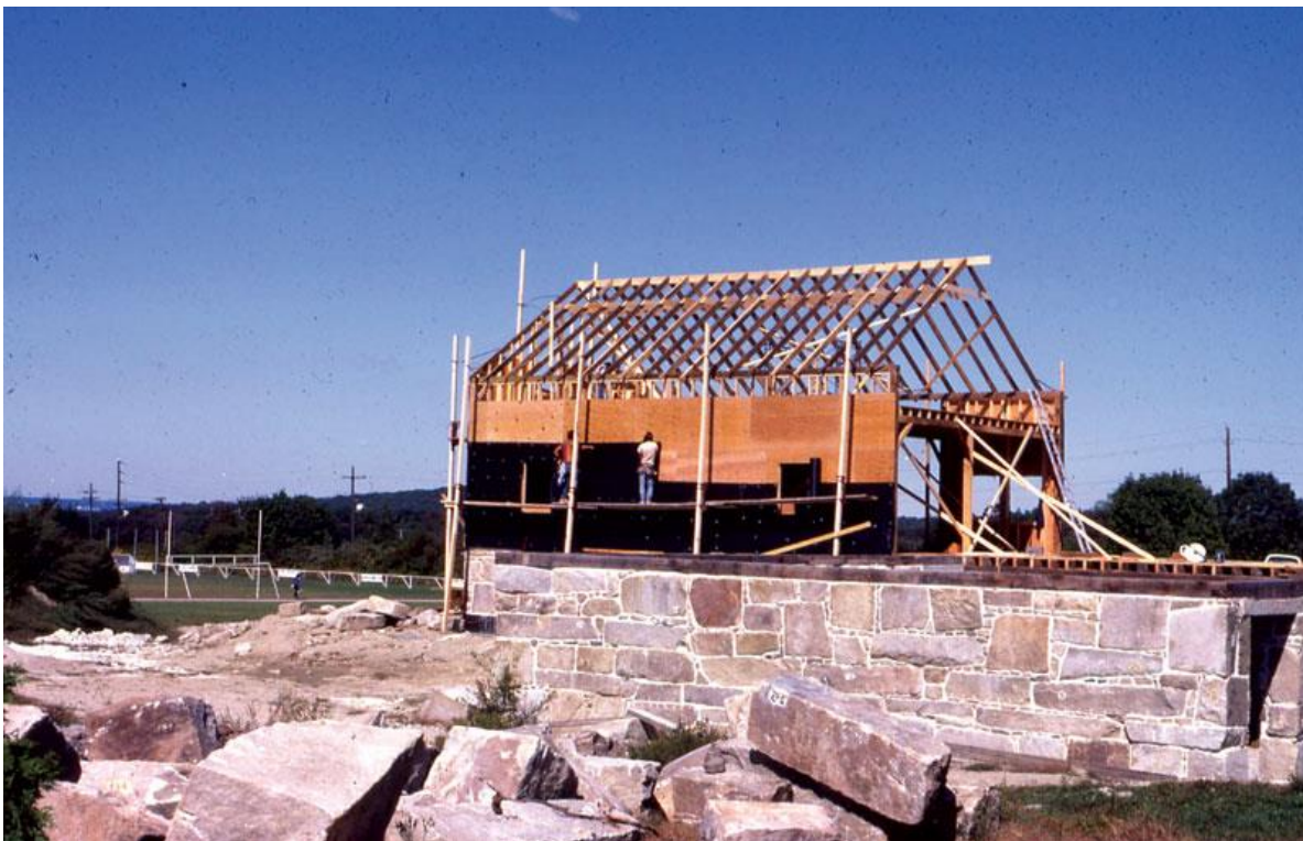
Plywood sheathing was applied to the sides of both barns. Here, the smaller barn takes shape.
